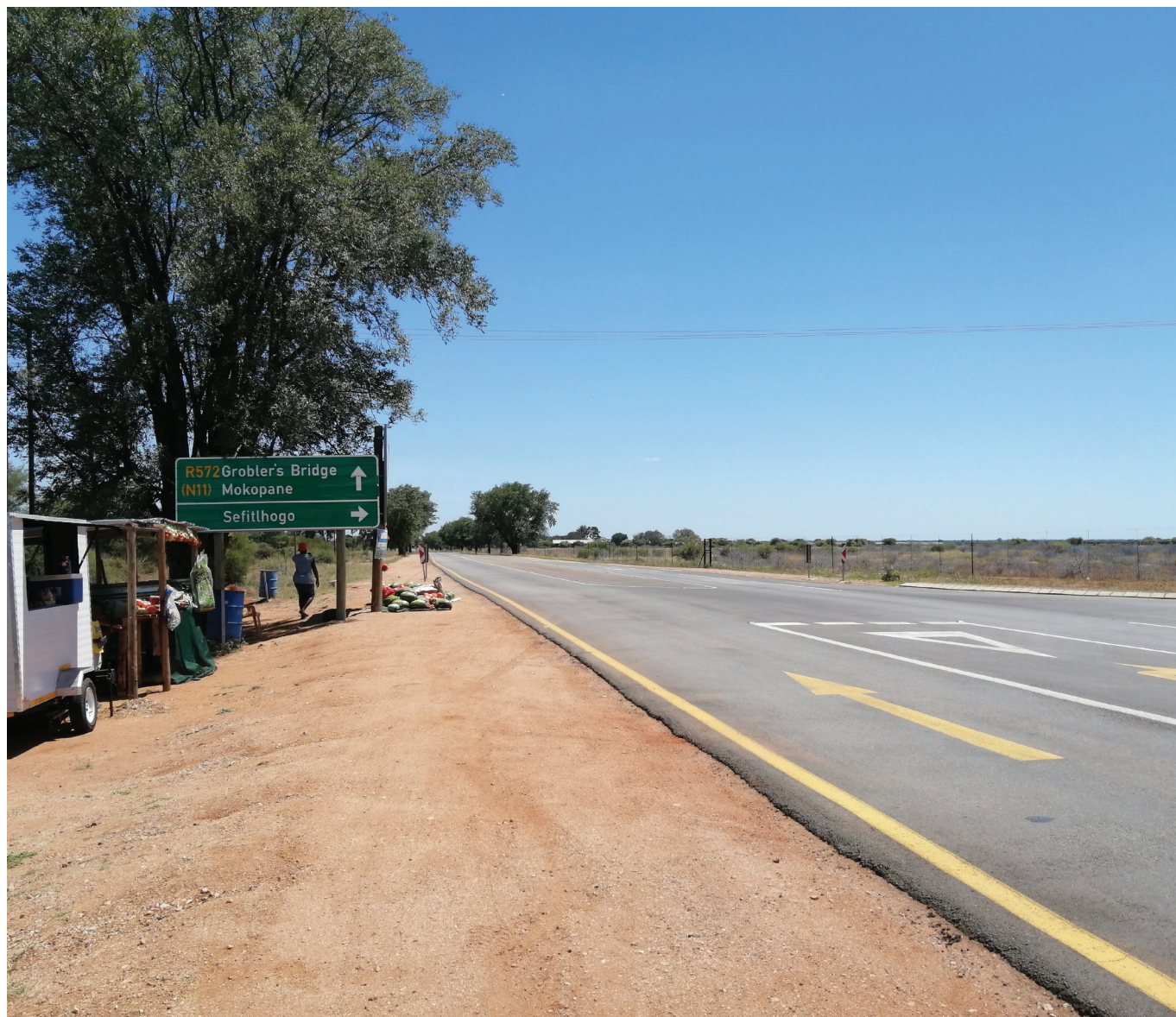
Road upgrade at Ga-Seleka in Limpopo
